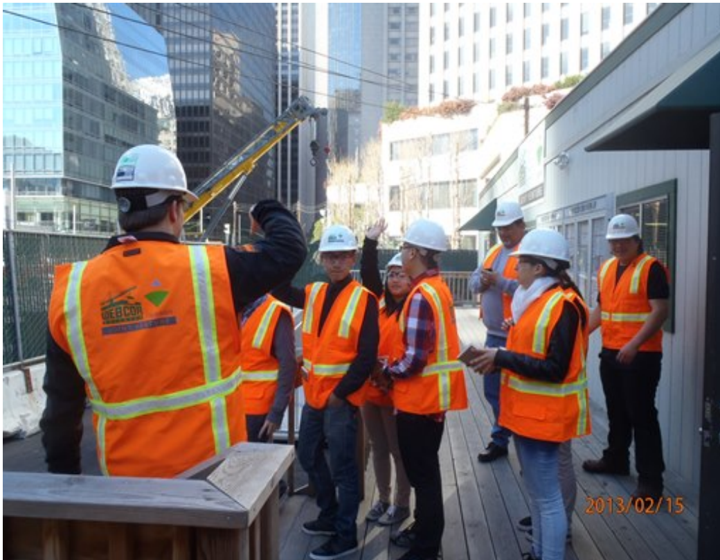
Students from the Tech 21 program get ready to tour the Transbay Transit Center construction site.
