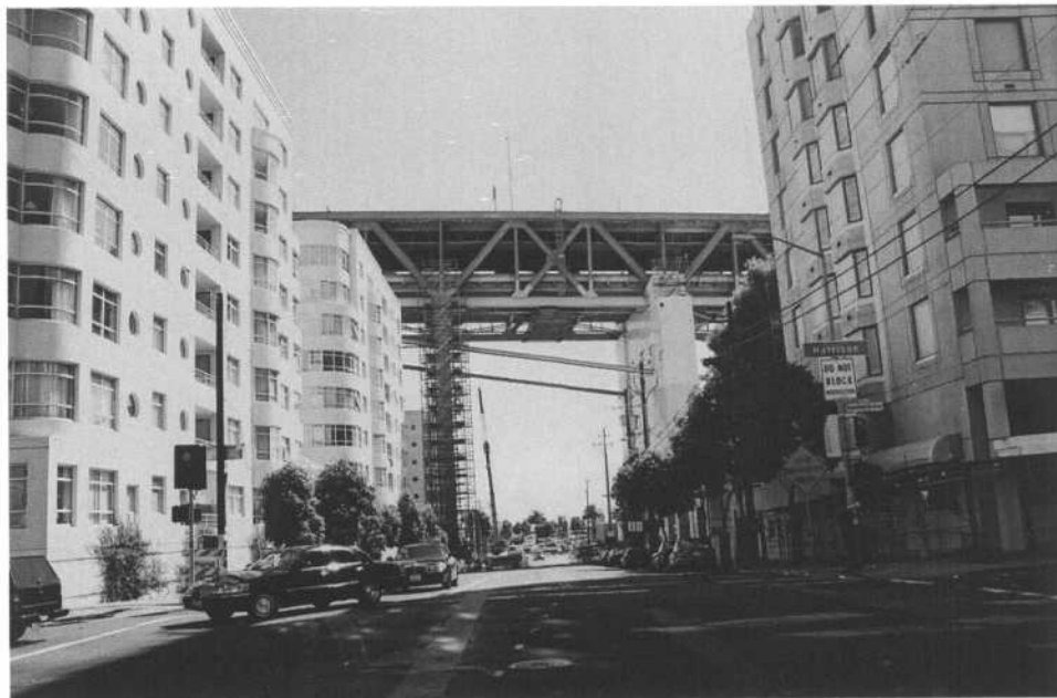
Fig 3B Beale Street, Looking South to Bay Bridge Steel Work
