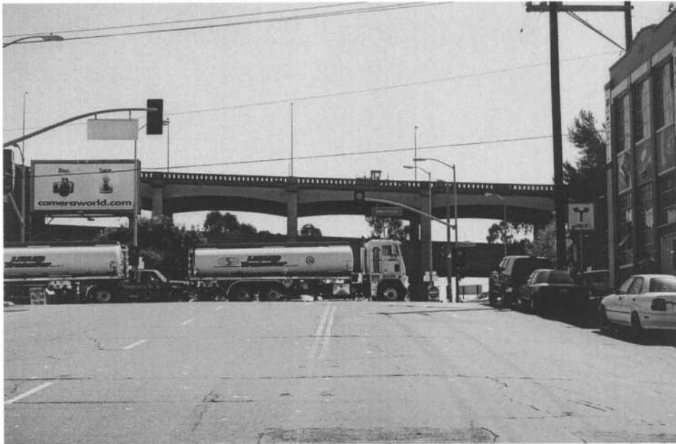
Fig 3A First Street, Near Harrison Street, Looking South to Elevated Bay Bridge Approach
