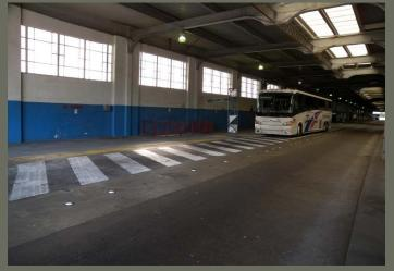
Transbay Terminal Bus Deck-Asbestos Skim Coat on Wall
